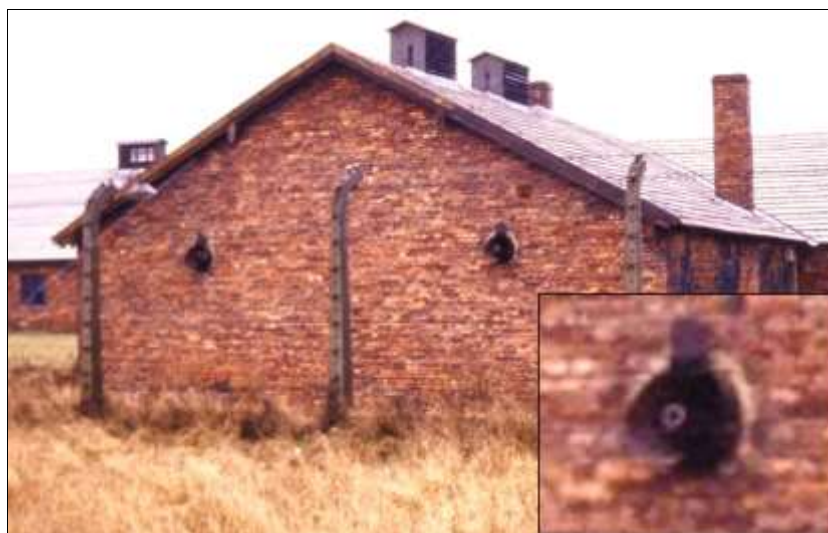
Auschwitz-Birkenau, inmates shower and disinfestation facility BW 5b, here the wing with the Zyklon-B fumigation chamber. Note the two openings for two air-extraction fans (now removed). Enlarged in the inset. (Photo of 1991.)
